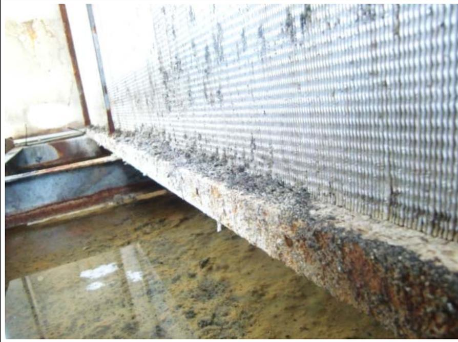
After a few short years when the condensate pan in your HVAC system becomes corroded and surfaces become irregular, troublesome leaks start.
