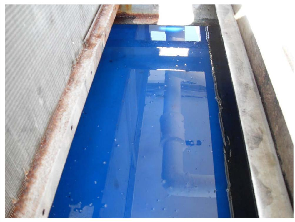
Pancrete automatically fills in pits and irregular surface characteristics, providing a smooth, enamel surface that is unaffected by harsh coil cleaners.
