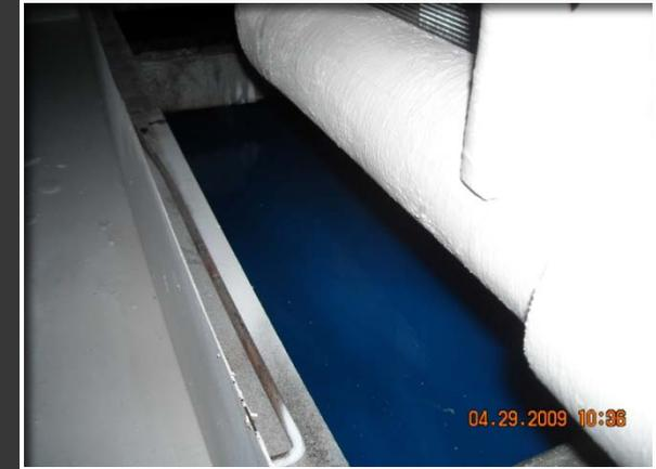
New condensate pans should be coated to remove dead spots on the pan surfaces, and protect the pan's surface from corroding. Applying Pancrete to a new pan will extend the life of the pan dramatically and perform better than a factory installed original galvanized pan.
